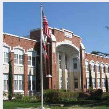
San Mateo High School is one of seven high schools and several other buildings in California's San Mateo Union High School District.
